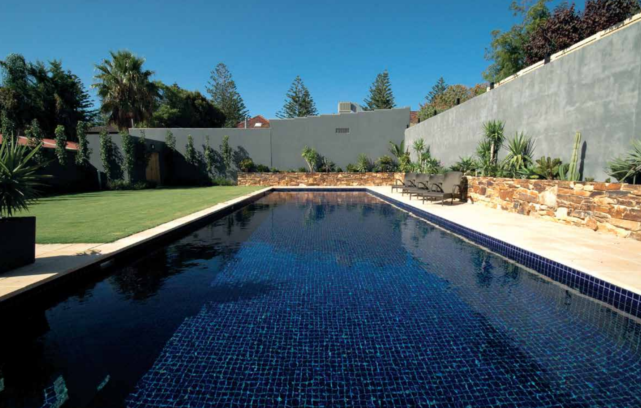
PROJECT: PRIVATE HOUSE, AUSTRALIA PRODUCT: MT 22S BL 15/R
